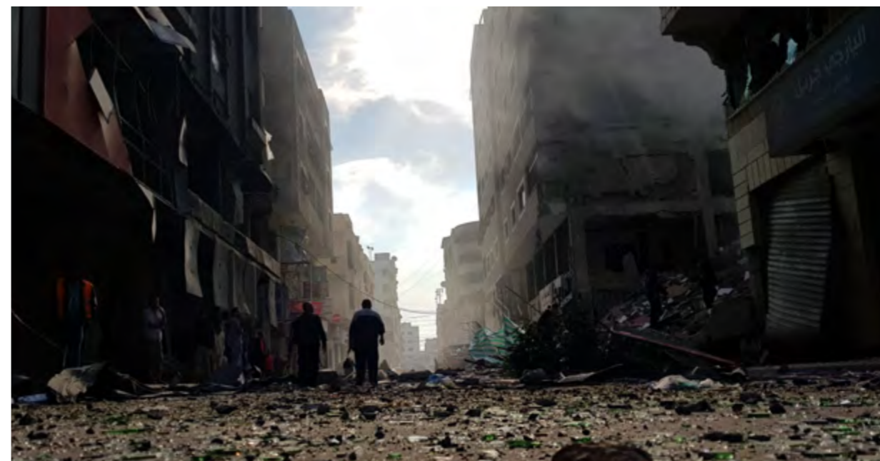
A scene of devastation after a residential multi-story building was targeted in the city of Gaza in the occupied Palestinian territory. Credit: Muthana El Najjar
